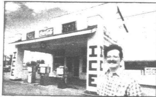
Quaint and comfortable, the Dennis Market on Canton Center Road dates to 1928 when grocer Colburn V. Dennis' father constructed it.
