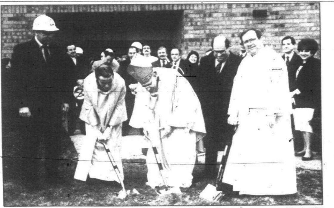
Groundbreaking ceremonies were held Sunday, Jan. 5, at St. John Neumann Catholic Church in Canton.
